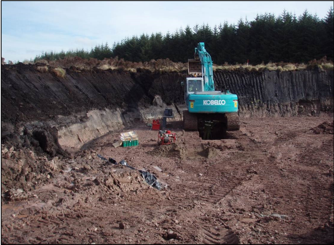
Figure 7-2 Excavation trimmed back to a stable temporary side slope
